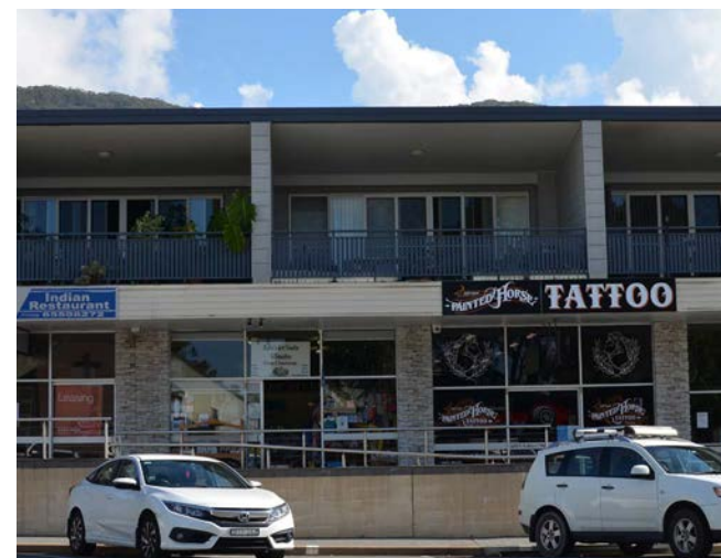
Figure 040. Shoptop housing along Bold Street
