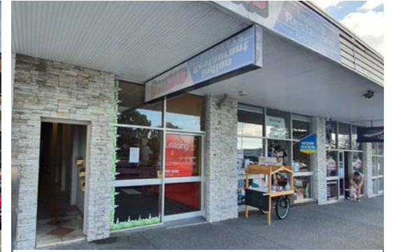
Figure 017. Bold street's evidence of vacant sites
