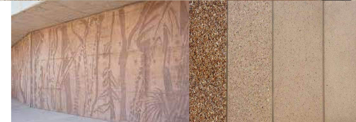
Angled sea wall with natural gelyogy matching oxide and sandblast designs
