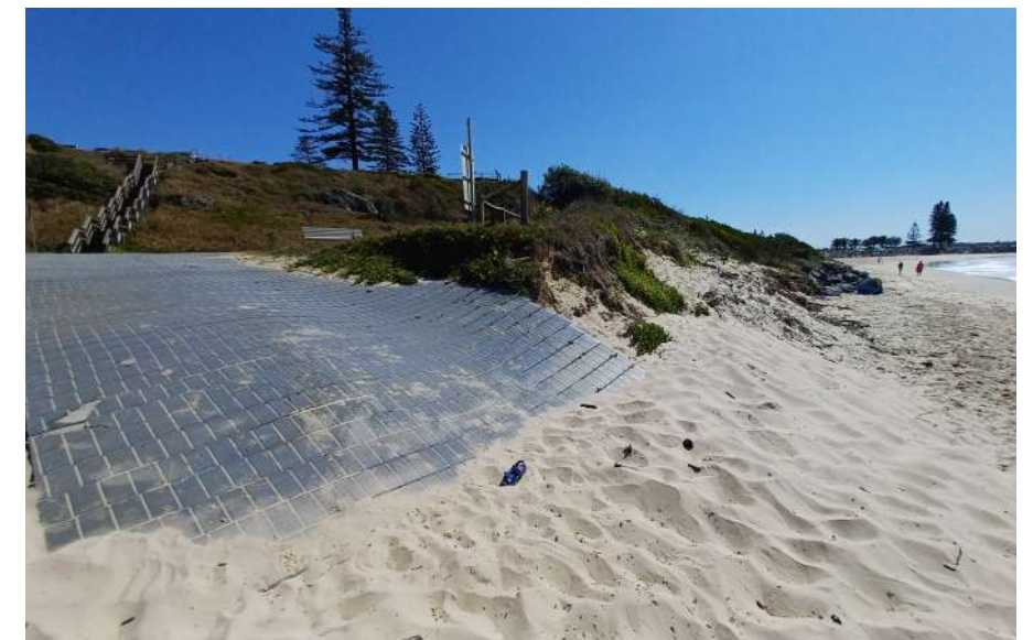
Ramp and foredune undermined
